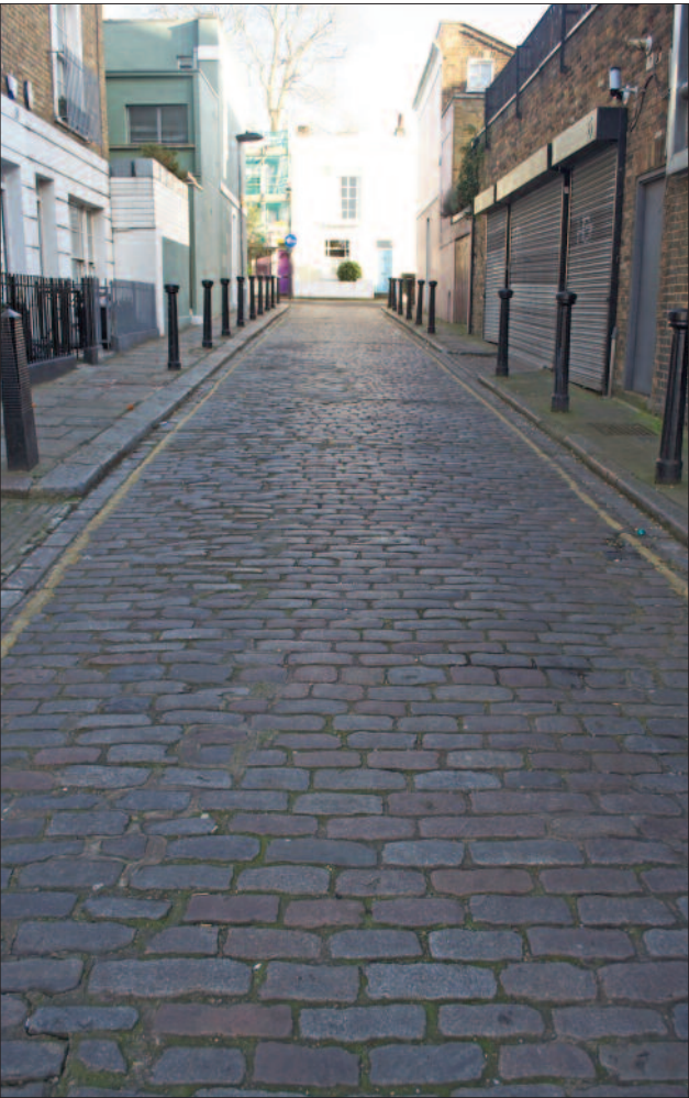
▲ Leverton Place, NW5 2PL, is a rare example of virtually intact and continuous granite setted carriage way. Continuity is broken only by some patching and a break where it intersects with Leverton Street. The high quality of setts, gutters and kerbs creates a consistency of setting for the variety of building types in this lane.
